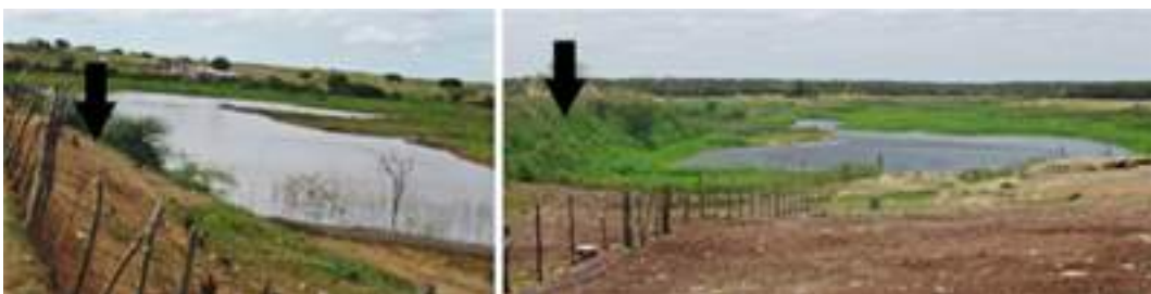
Fig. 9 Water tanks ( Barreiro ), the arrows indicate the earth bus that allows the accumulation of water. Record in the surroundings of the Poçoões community, in the Paraíba River basin, semiarid region of Brazil
